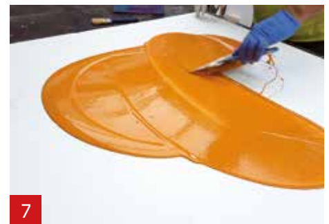
7 Apply a thin layer of A1 on the EPS with a spatula.
