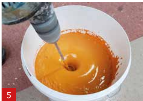
5 Stir for 1 minut until you have a smooth surface.
