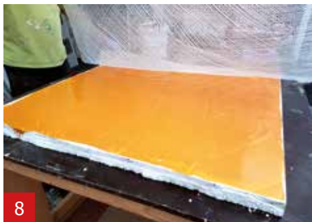
8 While still wet directly apply a piece of \pm 1 \text{ m}^2 triaxial fibre on the A1.
