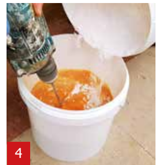
4 Add the A1 powder to the A1 liquid.
